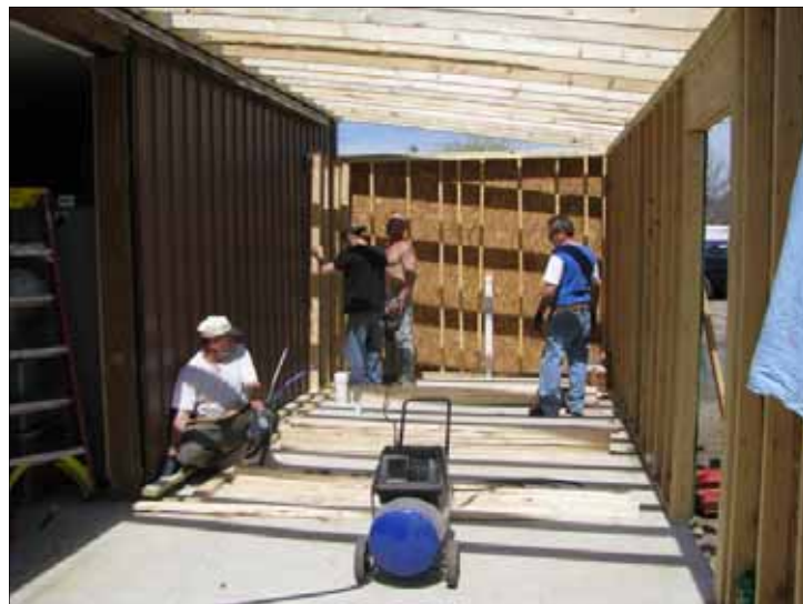
The new addition to the shelter under construction.
